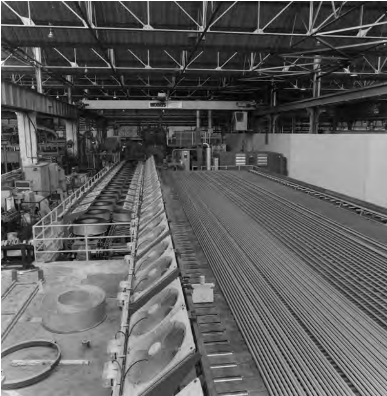
Fig. 6.59 Axial fans for wire coils in baskets
