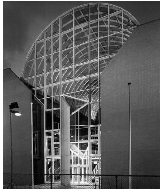
Fig. 2.60 Aluminum glass façade in combination with an illuminated courtyard and curved roof over the entrance of the Euro-Cetus-Complex in Amsterdam, Netherlands. Source: Hueck
