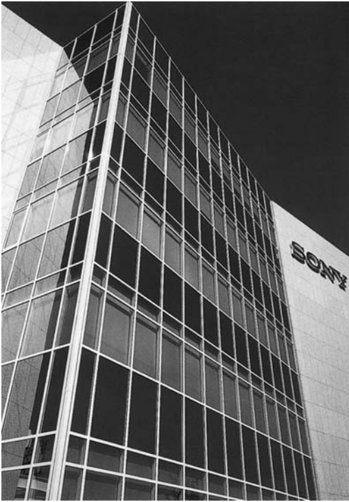
Fig. 2.58 Aluminum glass façade of a commercial building. Source: Hueck
