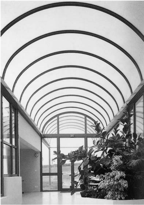
Fig. 2.61 Curved glass roof with aluminum sections for an illuminated courtyard of a sports center in France. Source: Cintro Systems
