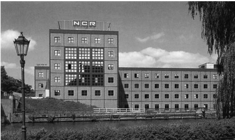
Fig. 2.63 Refurbishment of the NCR at Spree-Ufer in Berlin, Germany, with the blue baked painted aluminum window frames
