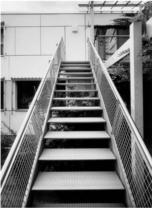
Fig. 2.71 Industrial stairs manufactured in extruded aluminum sections including those shown in Fig. 2.72. Source: Alusuisse
