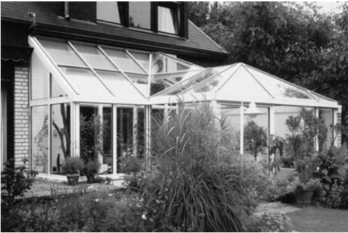
Fig. 2.67 Conservatory extension in extruded and thermally broken aluminum sections. Source: Sykon-Systems
