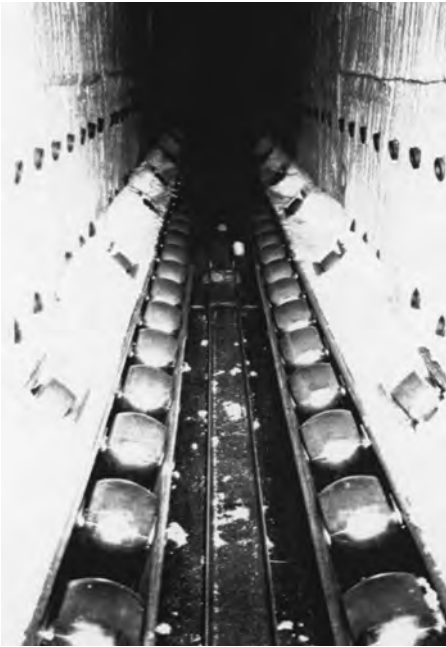
Fig. 6.53 Rapid-heating gas-fired furnace with transport rolls
