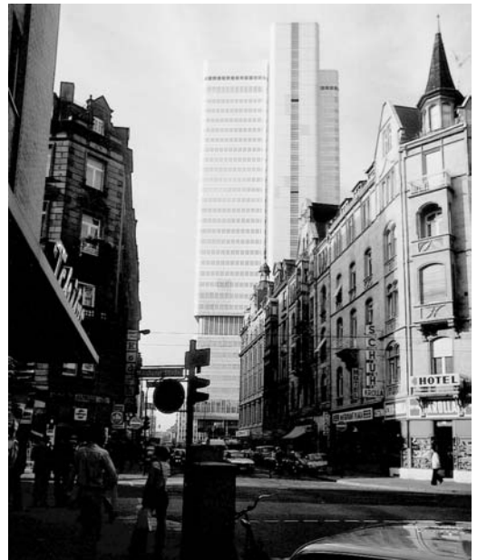
Fig. 2.57 Skyscraper of the Dresdner Bank in Frankfurt, Germany, with a naturally anodized aluminum façade
