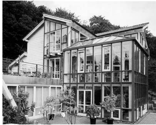
Fig. 2.68 House with conservatory-type construction based on aluminum extruded sections. Source: Sykon-Systems
